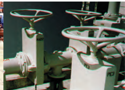
Fully closed, the Series 75 ensures drop-tight, bi-directional shutoff and an intrinsically safe design with no packing to maintain.
